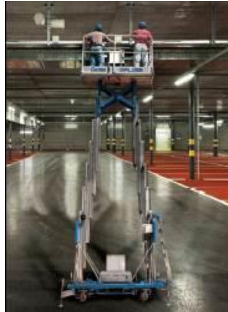
2-man Aerial Work Platform – effective work
