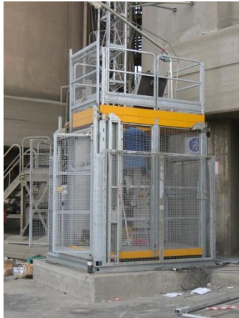
Passenger hoist in use without interfering with existing building daily operations
