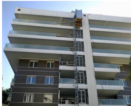
Passenger hoist in use without interfering with existing building daily operations
