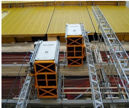
Passenger hoist in use without interfering with existing building daily operations
