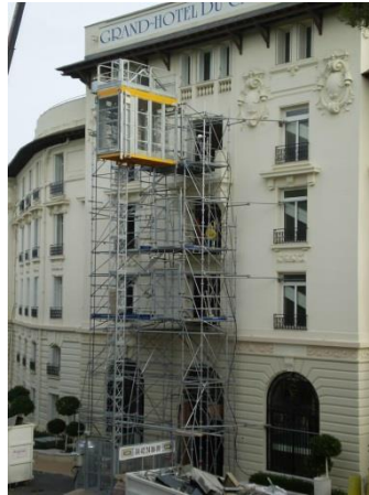
Passenger hoist in use without interfering with existing building daily operations
